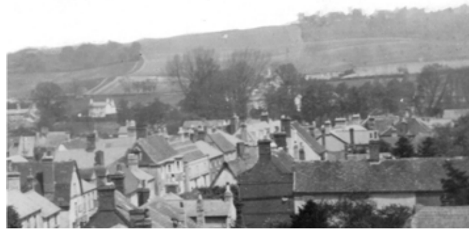
Greenhill Farm around 1907, the pair of C17 th cottages with dormer windows which were the original farmhouse can be seen on the left.
