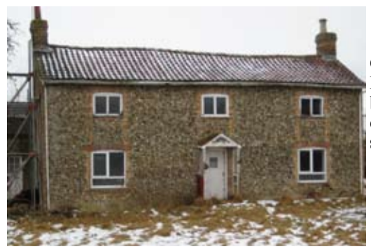
Greenditch Farm building in its current sorry state
