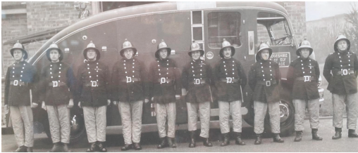
The original crew of the new Linton Fire Station
