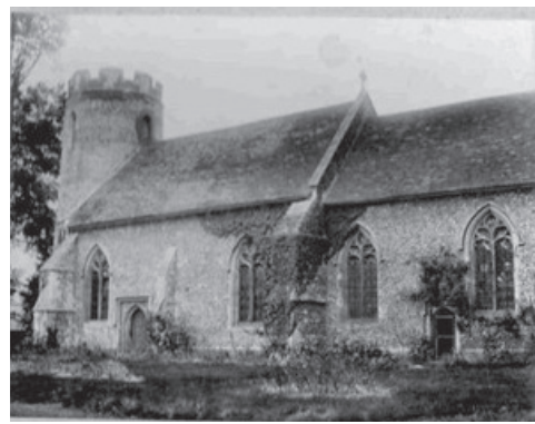
St Mary's Church Bartlow
