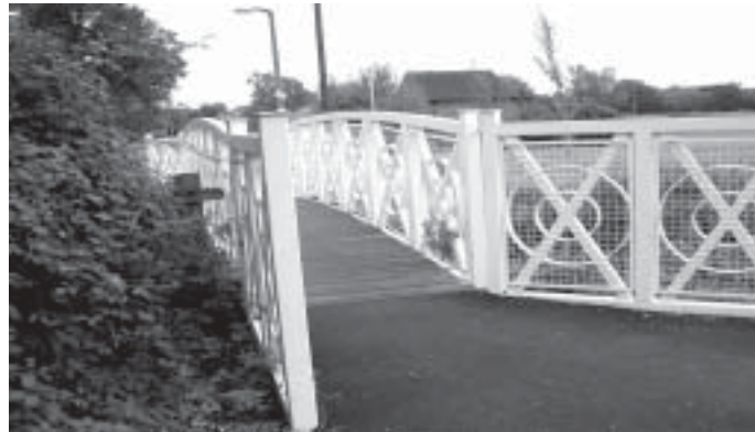
Stantons Lane Bridge
