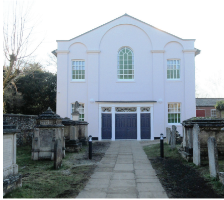
A new coat of paint on the front, but the real magic is inside
