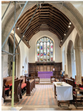
The last of the scaffolding coming down at St. Mary's
