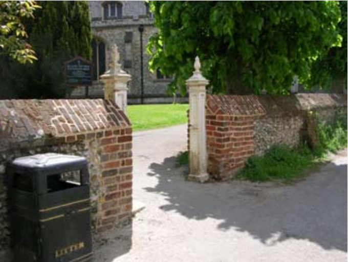
Rebuilt piers at the main entrance gate to St Mary's church
