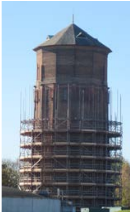
The scaffolding goes up
